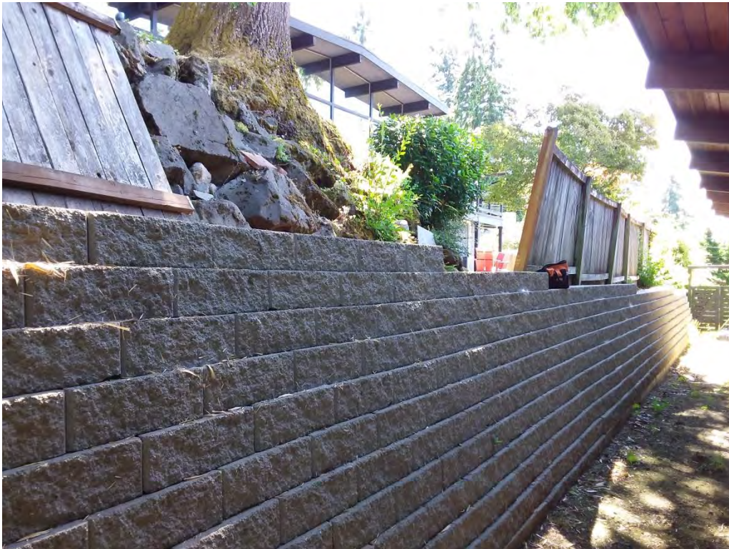
Figure 8. Looking SSE down the length of the Keystone block retaining wall running along the east side of the existing house. Note the base of the #5 oak at top center of the photo, The edge of the existing roof is visible in the top right corner of the image.
