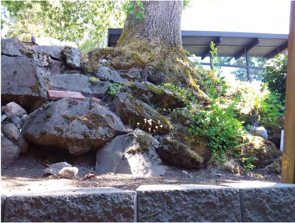
Figure 7. Looking up and east at the base of the #5 oak. The concrete blocks at the bottom of the photo are the top or the Keystone wall shown in Figure 8.
